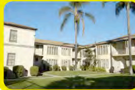
Existing residential neighborhood in Crenshaw
